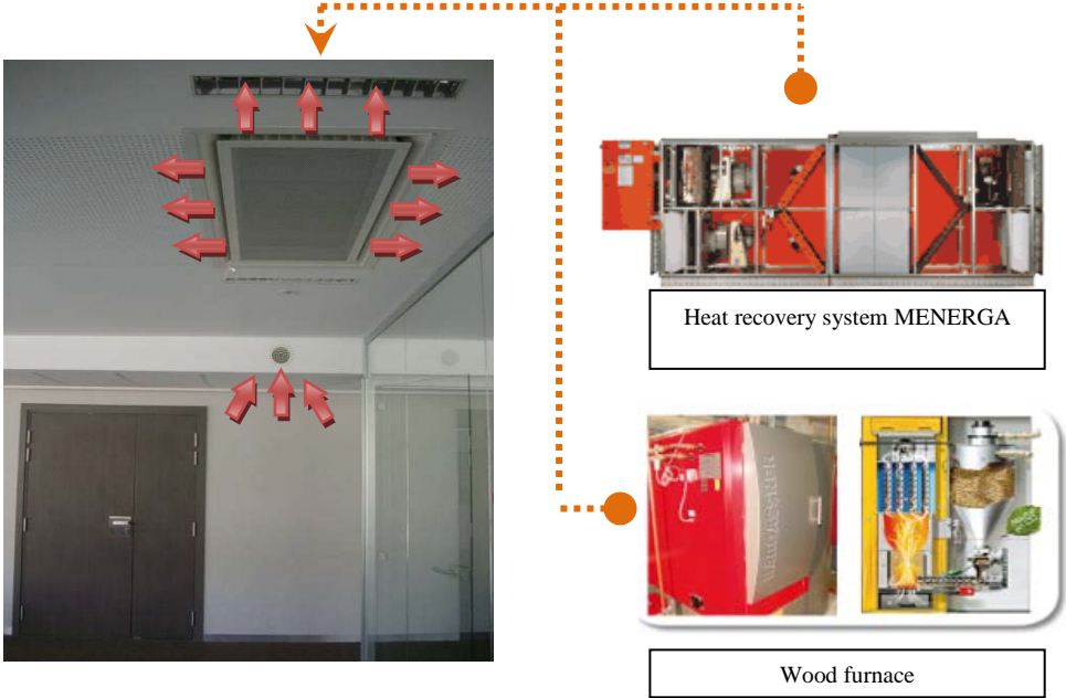
Figure 7. Air Distribution - cold beams
