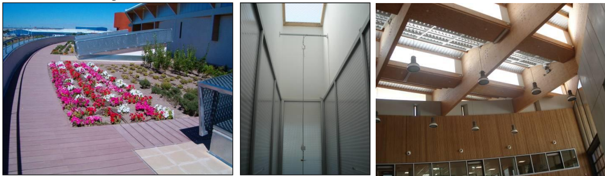
Figure 2: Passive and active strategies. From left to right: gardened roof, lucernaire and central atrium
