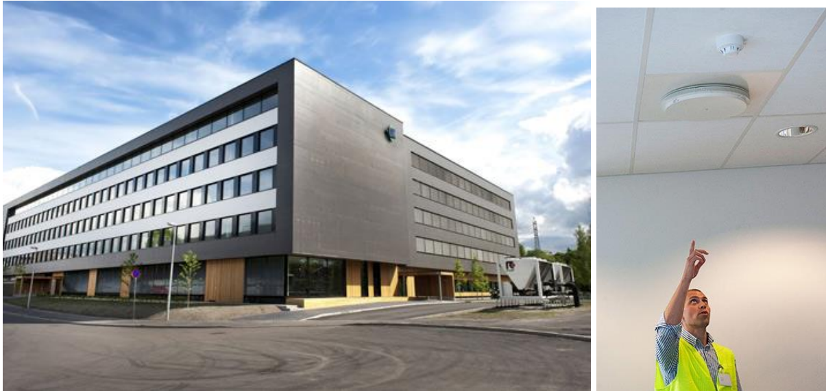
Figure 1: The GK Environmental house and the active air supply diffuser used
