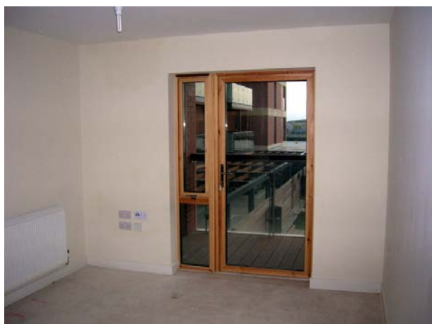
(a) Photograph taken of balcony doors in living room of test flat at time of thermographic survey
