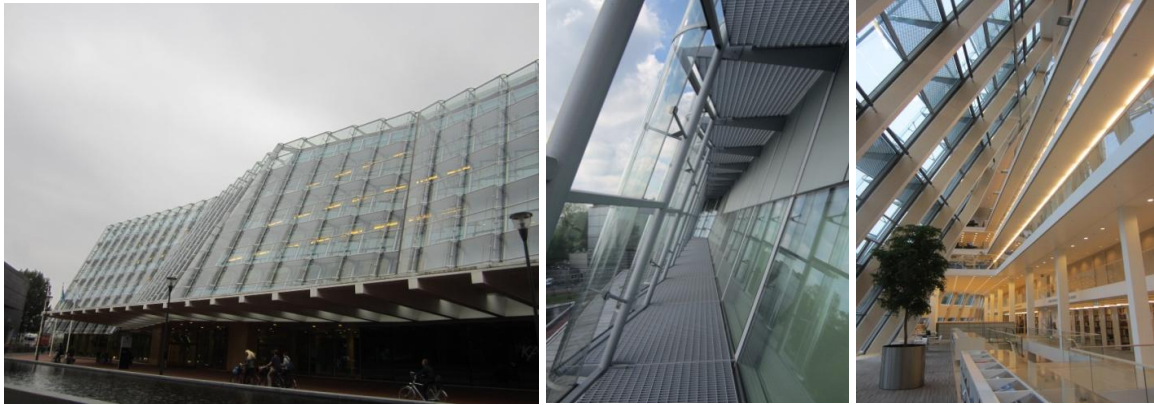
Figure 1: Outside of the façade, the cavity of the DSF and the atrium behind the DSF
