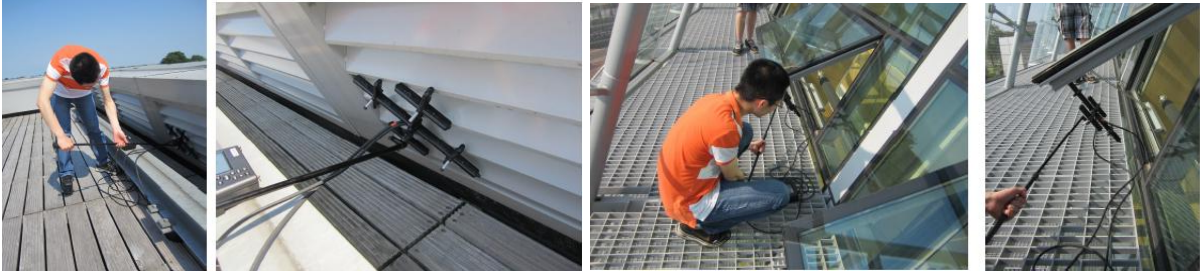
Figure 4. Measurements of air quantities at roof outlets and inlet windows on 4 th floor
