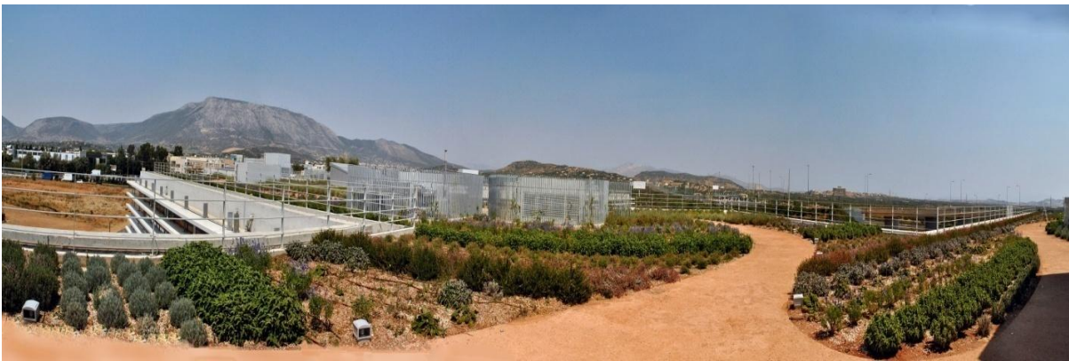
Figure 3: A panoramic view of a part of the green roof
