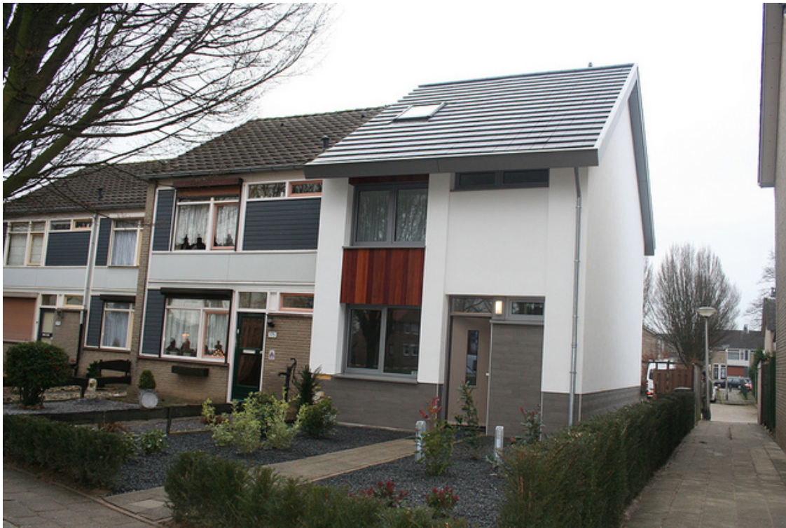
Example of a renovated dwelling in Kerkrade, Energyleap programma P31 (picture: Frank Hanswijk, Platform31)
