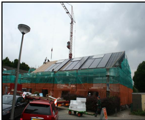
Finishing zinc en roof trims
