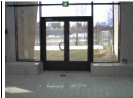
Figure 8. Entrance door of pool unit
