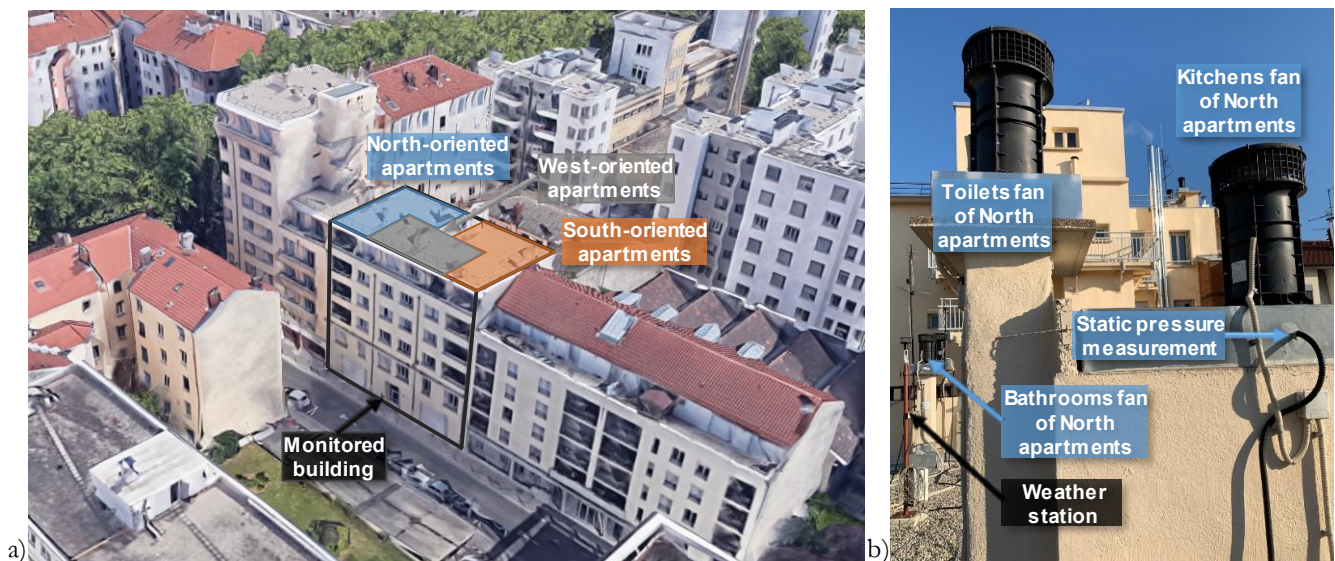
Figure 1 (a) View of the west façade of the monitored five-level multi-family apartment building and (b) view of the assistance fans of the north-oriented apartments located on the roof.
