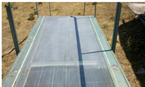
Figure 2: Closer look to the glass above the panels
