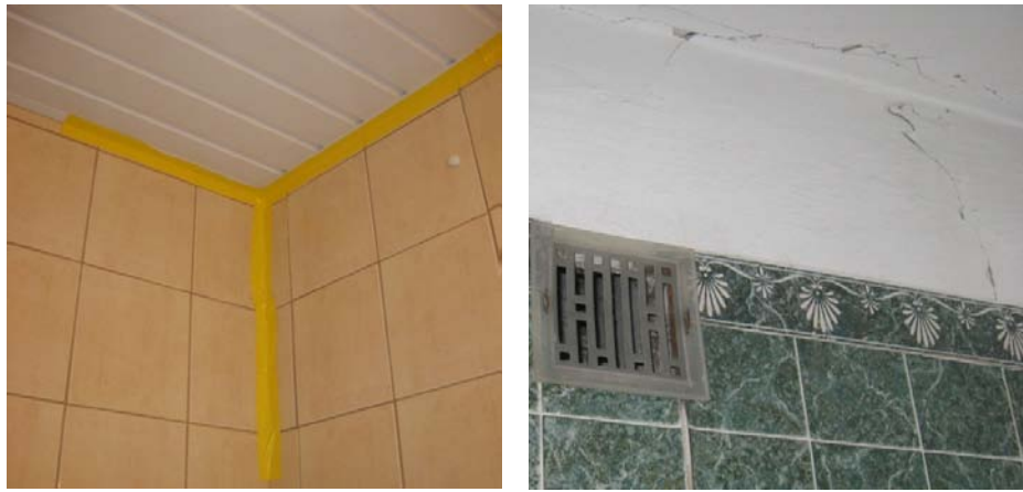
Figure. 2. The examples of leakages in the walls and ceiling of the apartments
