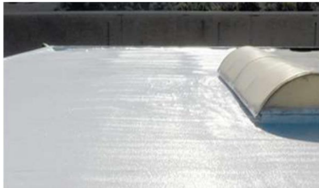
Figure 1 Example of roof application of the developed material that will be applied in Cadiz, Source: INDEX Construction Systems and Products Spa
