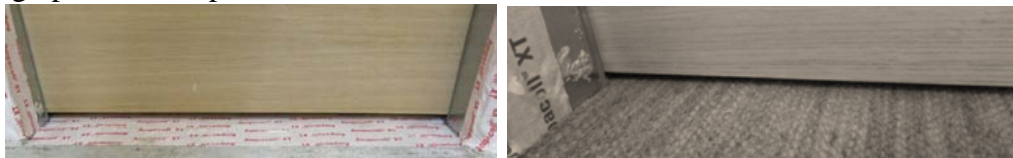
Figure 7: Measured door gap without (left) and with carpet (right).
