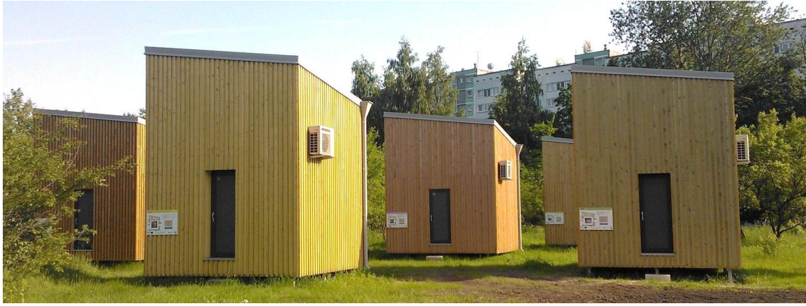
Figure 1: Experimental test buildings
