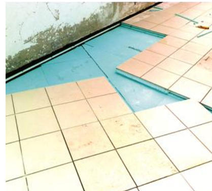
Figure 5: Retrofit insulation on Flat Roof
