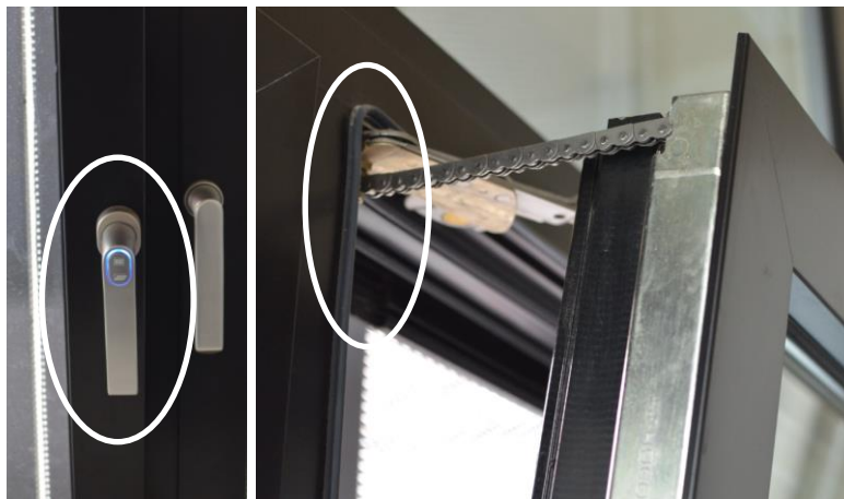
Figure 8 Automated window, with optional manual operation and resistance sensitive gasket
