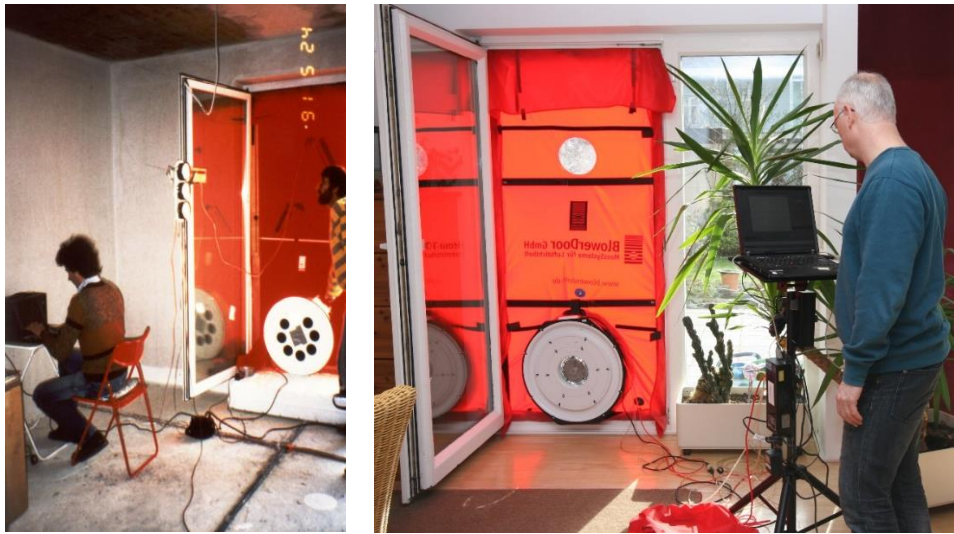
Figure 4: Left : The first pressure test was conducted on 24/26 of May 1991 by Ingenieurbüro ebök once the airtight envelope had been finished. Right : The current Blower Door Test (here in House B) was conducted on 11/12 of February 2016 by the PHI 25 years after construction.
