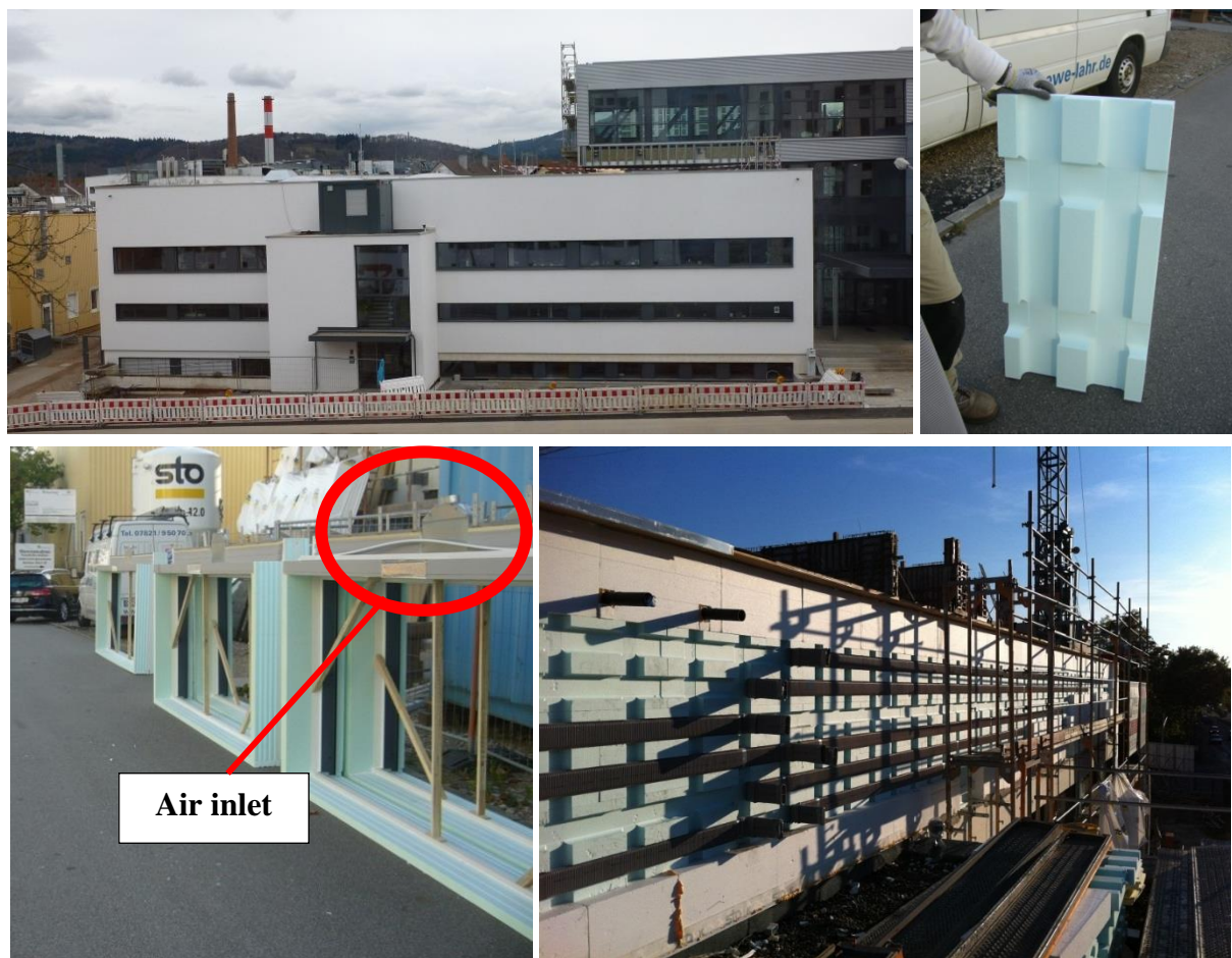
Figure 1 Retrofitted façade of the demonstration building and retrofit concept
