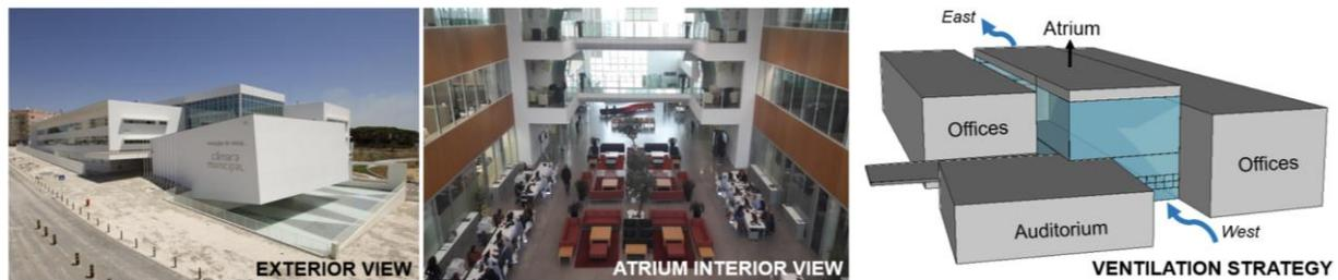
Figure 1 Building view from the outside (left), an internal view of the central atrium (middle) and night ventilation strategy (right)
