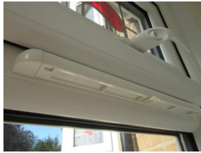
Figure 3 – Trickle vent closed
