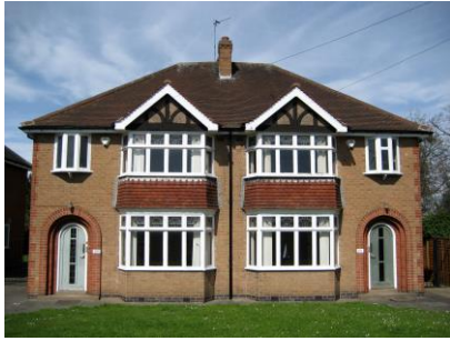
Figure 1 – Ashby Road Test Houses pre-refurbishment, only the left house was used
