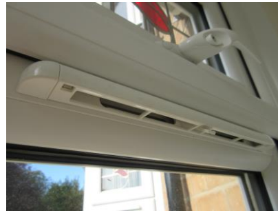
Figure 4 – Trickle vent open
