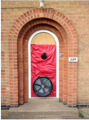
Figure 6 – Front door with a semi-circular wooden panel to fill the gap in the upper arch.
