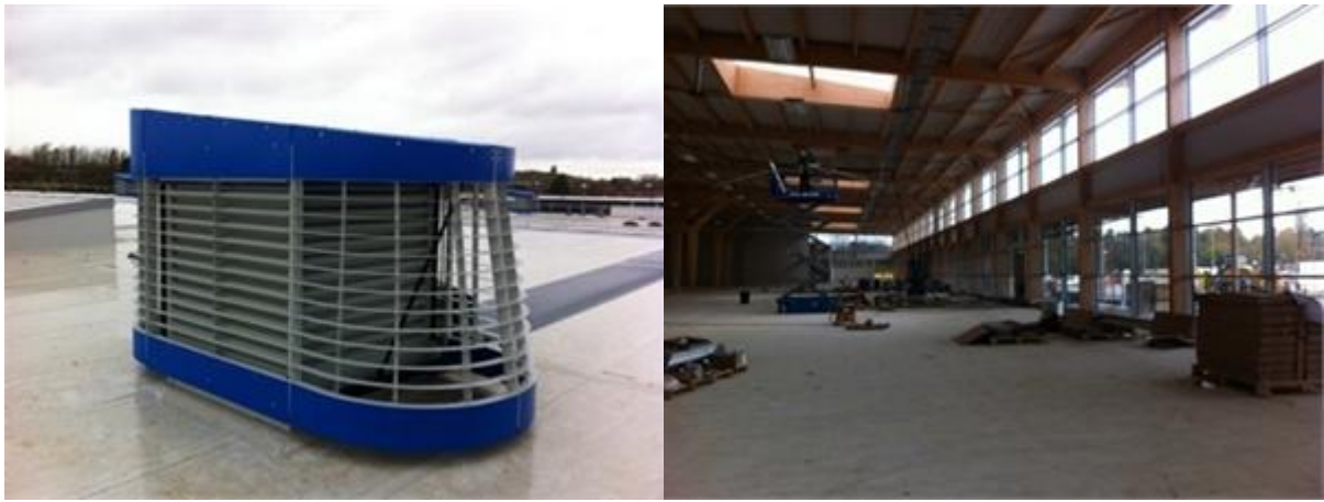
Figure 7: Windcatchers of a supermarket opened in January 2013 (courtesy of Monodraught Ltd).
