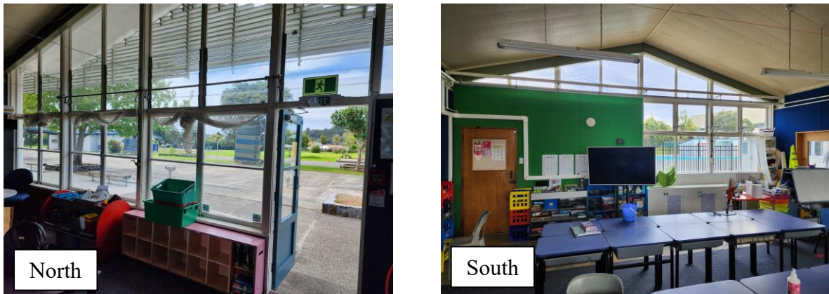
Figure 3: Design of windows in S0R2 and five other classrooms.
