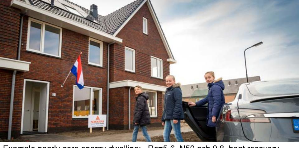
Example nearly zero energy dwelling: Rc=5-6, N50 ach 0.8, heat recovery, heat pump, PV -> can be built without subsidies
