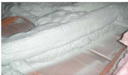
Figure 20. Ductwork well-sealed to sheetrock with ccSPF
