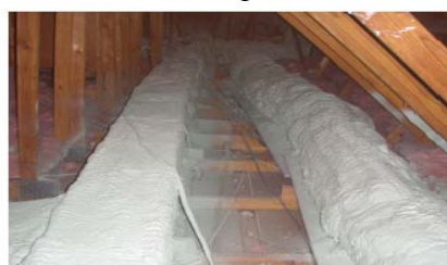
Figure 23. Varying application thicknesses shown on rectangular (left) and round (right) ducts
