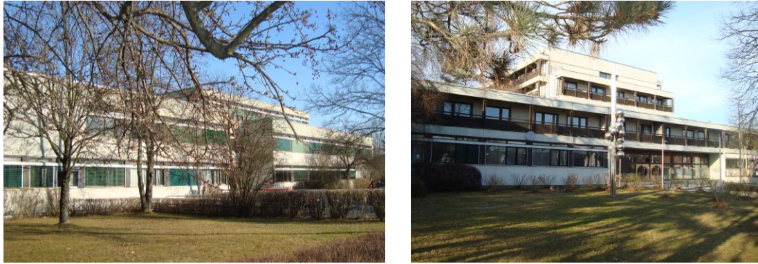
Figure 2: Views of the existing school building in Gleinstätten/Austria (Source: AEE INTEC)
