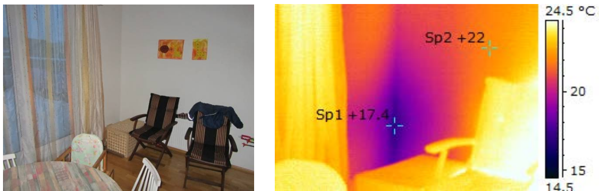
Figure 5. Air leakage between separating walls and the external wall.
