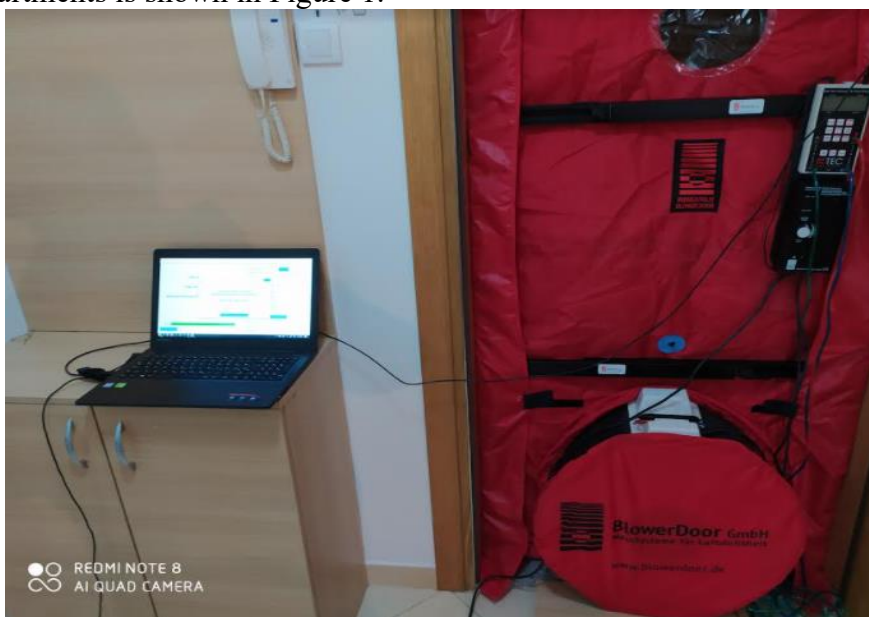
Figure 1: Blower door fan mounted on the front door of the apartment
