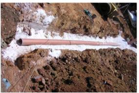
Figure 5: Placement of a pipe into the ground using sand to improve thermal contact between the pipe and the soil
