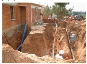
Figure 4: Placement of a pipe into the ground
