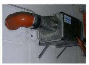
Figure 9: Point where the air from the earth tube is introduced in the building
