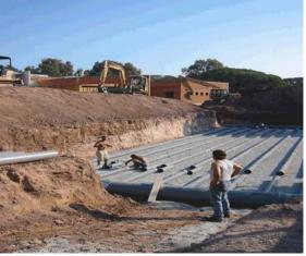
Figure 6: Buried pipes with a common inlet and exit [Ref. 1]
