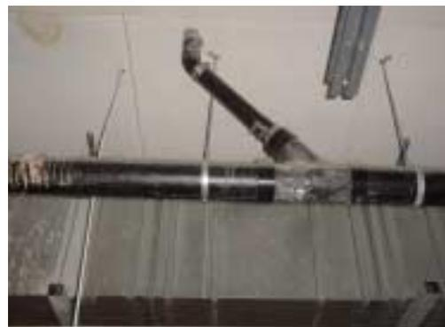
*Figure 81 : A rectangular duct has to be supported on both sides with hangers – compare with the pipe.*
