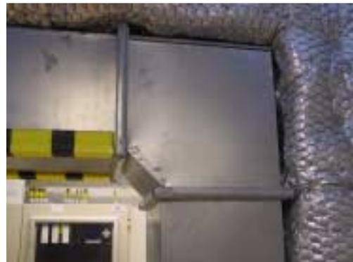
**Figure 71 : Slip joints on a rectangular bend**
