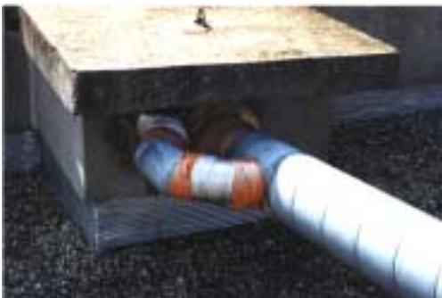
*Figure 118 : Branching between a flexible and a rigid duct.*
