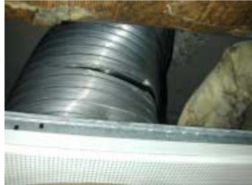
*Figure 119 : Leak found at a supply air terminal device.*
