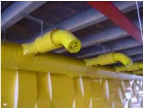
*Figure 106 : Close-up view of supply air register with sound silencer*
