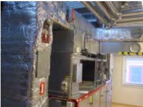
Figure 53 : Clean-out and inspection openings on vertical duct (left) and horizontal ducts.
