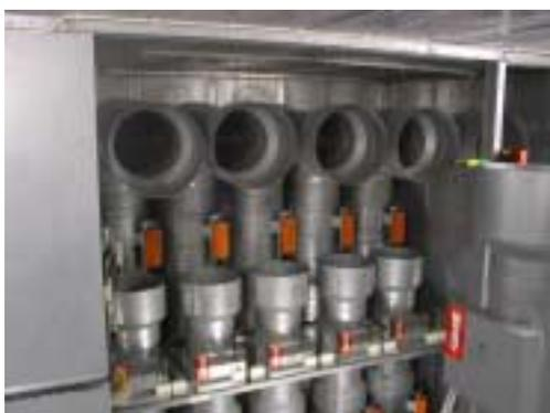
**Figure 103:** Ducts for the different floors pass down through common shafts, one for supply and one for extract air.
