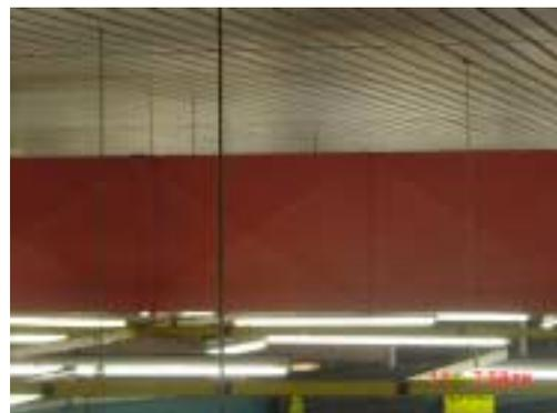
**Figure 72 : Cross-bent duct sides to increase stability.**
