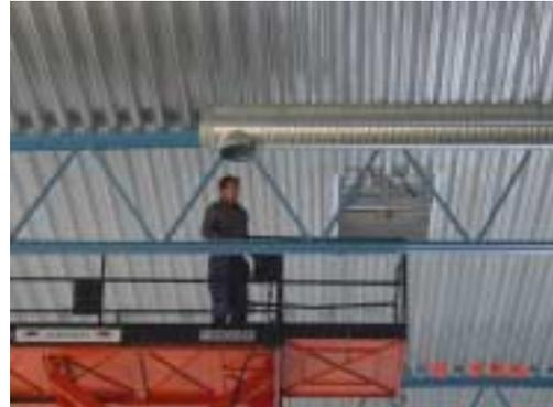
*Figure 79 : Installation of ductwork from a movable platform.*
