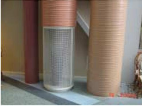
*Figure 111 : Supply air register*
