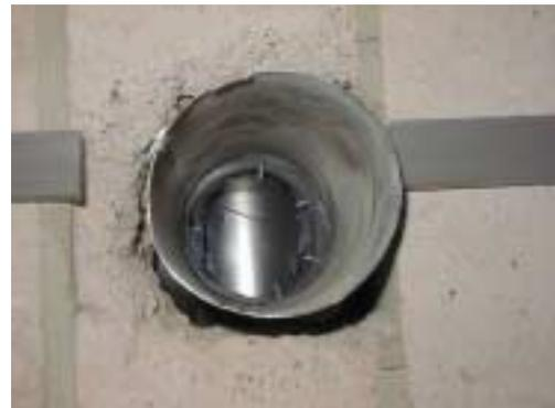
*Figure 120 : Sharp screws increase the risk of injuries during maintenance operations*
