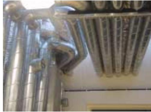
*Figure 100 : From the fan room the ducts are passing through the ceiling space to the rooms.*
