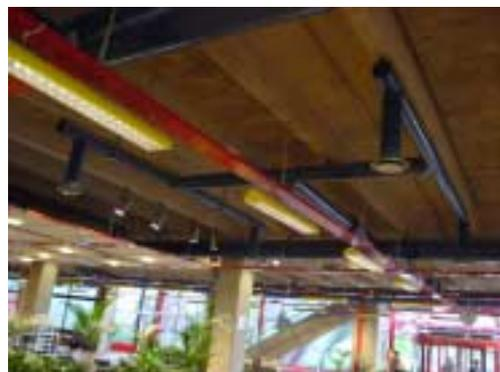
**Figure 20** You don't always have to hide the ducts. Here false ceiling (seen to the left) has only been used where needed for acoustical reasons.
