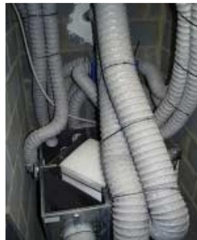
*Figure 116 : Inappropriate use of flexible ducts*
