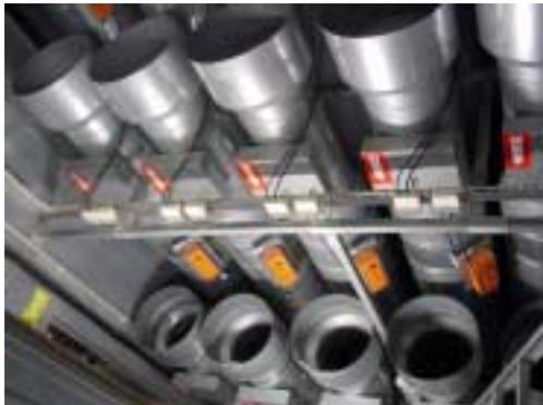
**Figure 41 : Installation of vertical ducts in a high rise building in a space saving manner.**
