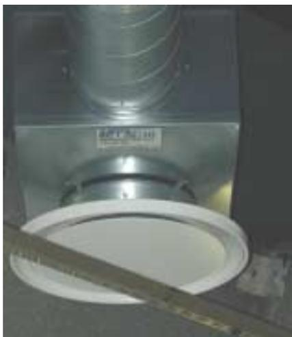
**Figure 16.** Plenum box connected to an air terminal device. Includes a regulating damper and acoustical cladding.
