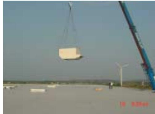
*Figure 33 : Large roof mounted air handling unit lifted by crane to its location*
