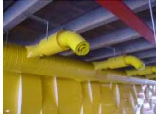
**Figure 39 :** Registers installed in parallel in a duct have to be provided with individual dampers, and perhaps also, as here, with silencers to reduce the noise from the dampers. Ducts (yellow) in a restaurant.
