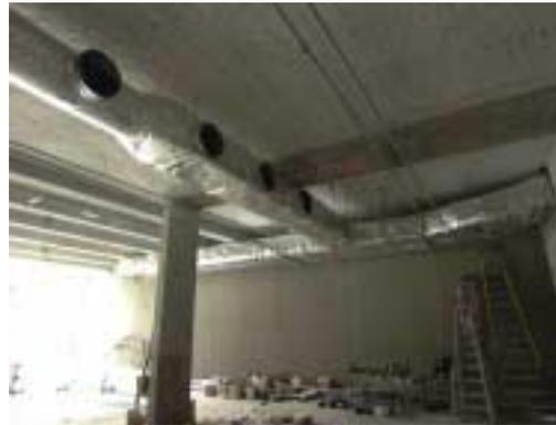
*Figure 114 : Rectangular to circular reducer*
