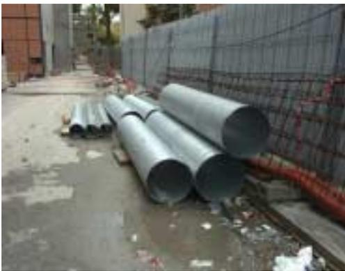
*Figure 112 : Ducts exposed outside on construction site.*
