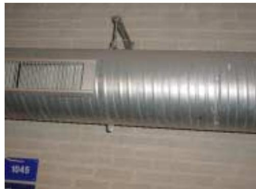
*Figure 80 : Bracket-hanger for circular duct.*
