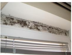
Figure 3: Left, new energy efficient and airtight windows in an uninsulated wall. Right, consequences of constant ventilation with window in an inclined position.
