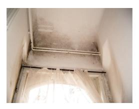
Figure 4: Mould growth on the bathroom ceiling, heating turned off, poor ventilation.
