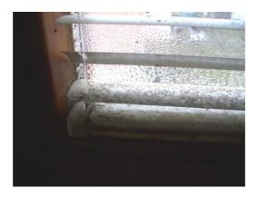
Figure 2: Condensate on glazing internal surface, and mould on internal blinds.
