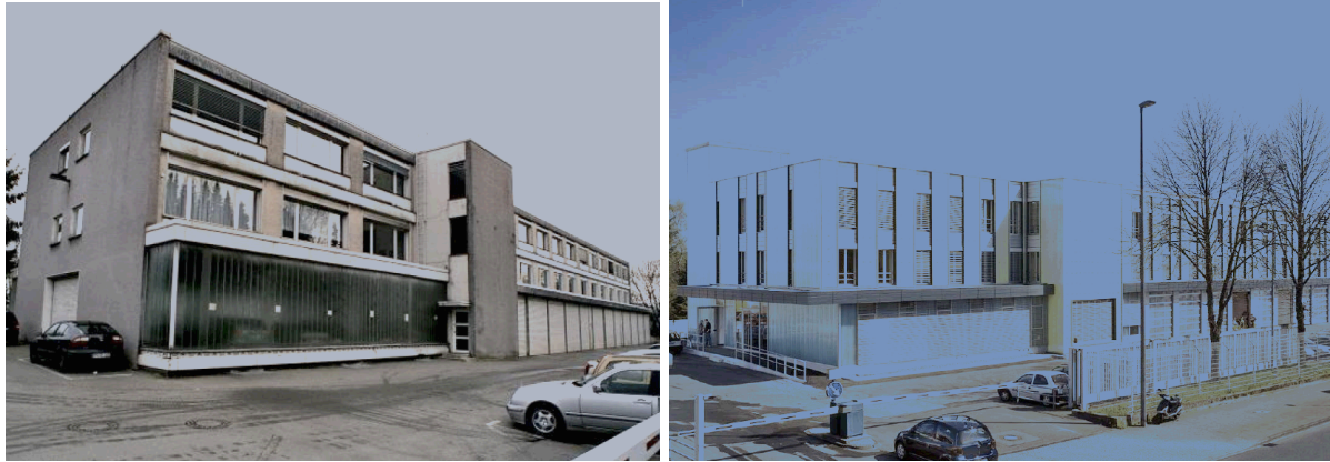
Fig. 1: Exterior view of the building before and after renovation. (Sources: l: [amcs], r: [Riehle])
