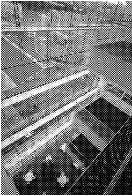
Figure 2: South side atrium
