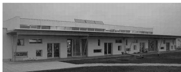
Figure 8 – Outside view of the Ziersdorf Kindergarten.
