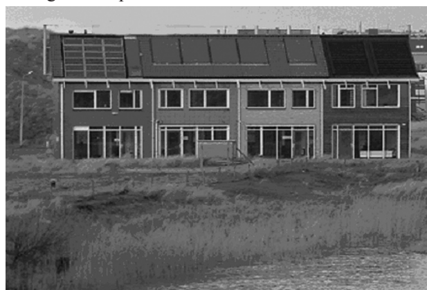
Figure 1: The four single-family research dwellings at the ECN premises. The second house from the left is used for these experiments.
