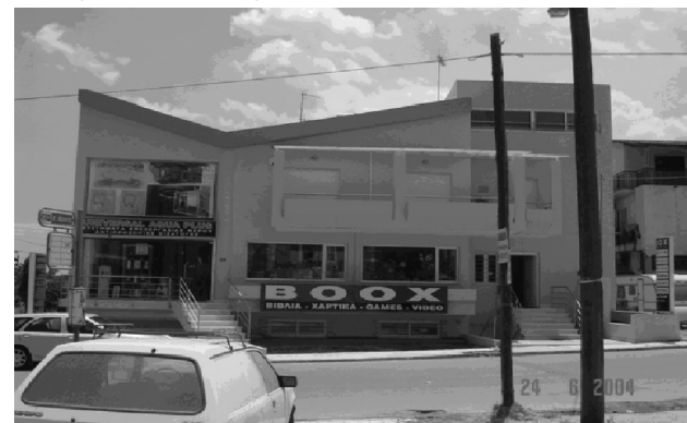
Figure 2: The building of application (Georgiadis, Athens).
