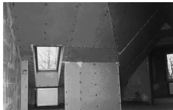
б) porous monolithic concrete in external walls and overlappings in a mansard floor
