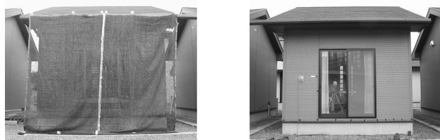
Photo 1: Two experimental buildings with radiative cooling (Bldg. RC, left) and convective cooling (Bldg. CC, right)
