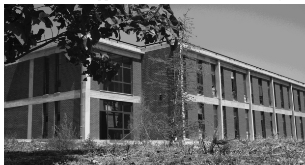
Figure 3. East (long) and south (short) façades of C Block
