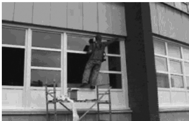
Figure 2 : Example of delicate posture while putting silicone sealant.
