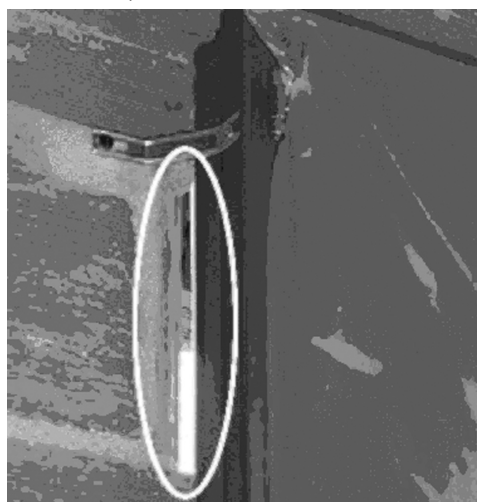
Figure 1 : Example of inadequate carcass work : opening size is too large given window size.
