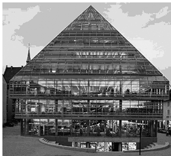
Figure 1. Example for a double skin façade building: The central library in Ulm, Germany.
