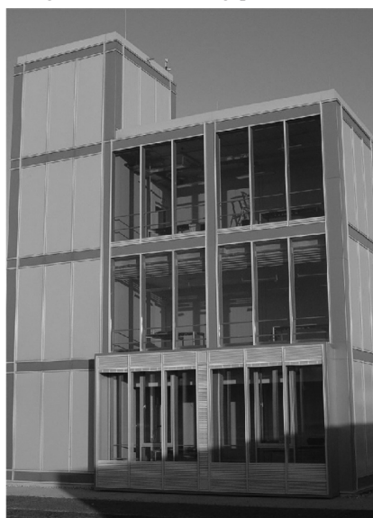
Figure 4. Photo of the test facility VERU in Holzkirchen, Germany.
