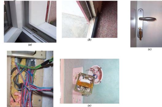
Figure 1. Examples of refurbishment measures. (a) replacement of windows. (b) Replacement of undercut joint and joint around the opening. (c) Replacement of the garage lock. (d) Injection of insulation foam to close the passageways to the air gap in the wall. (e) Insulation foam behind the plug boxes in cold walls.
