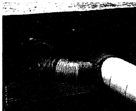
Figure 2: Photograph of poorly installed duct connections.
