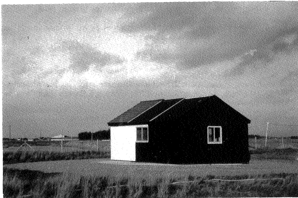
Figure 6 : View of the BOUIN experimental house
