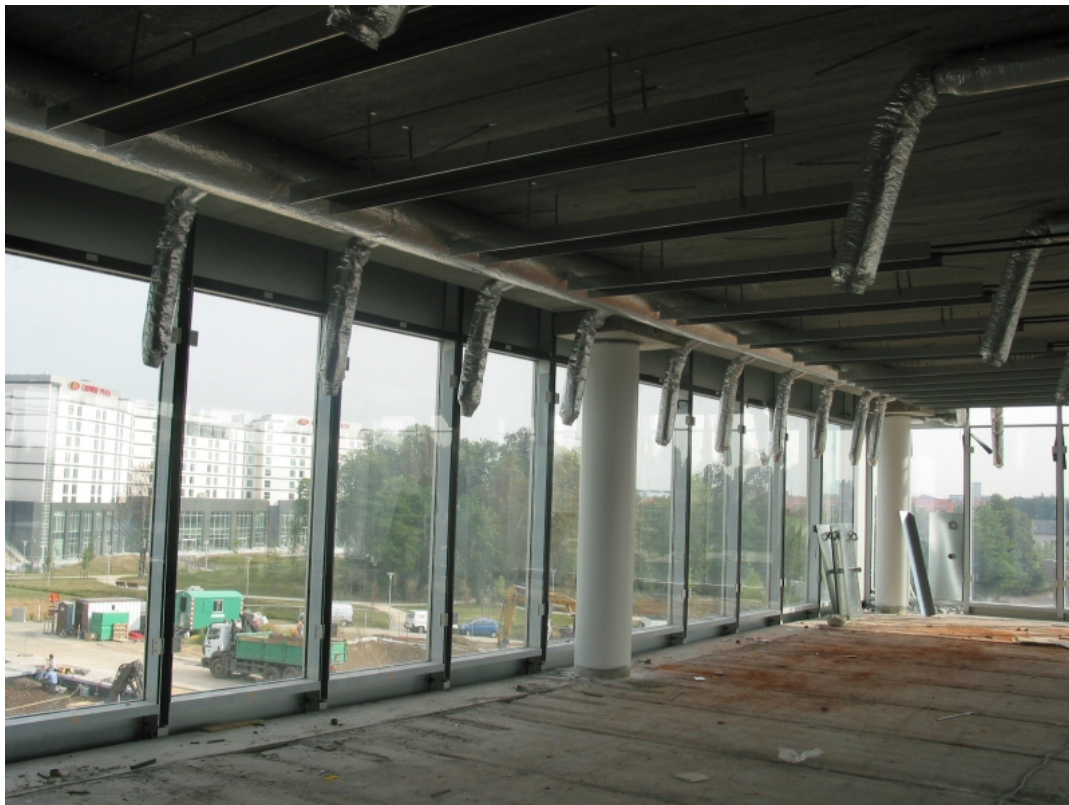
Fig. 16: View of installations combined with a mechanically ventilated double facade partitioned by storey with juxtaposed modules - View of the insulated supply ducts (in the upper right) - View of the insulated extraction ducts to be connected to the facade modules via the ventilation plenums located at the top of the facade elements - View of the cold beams
