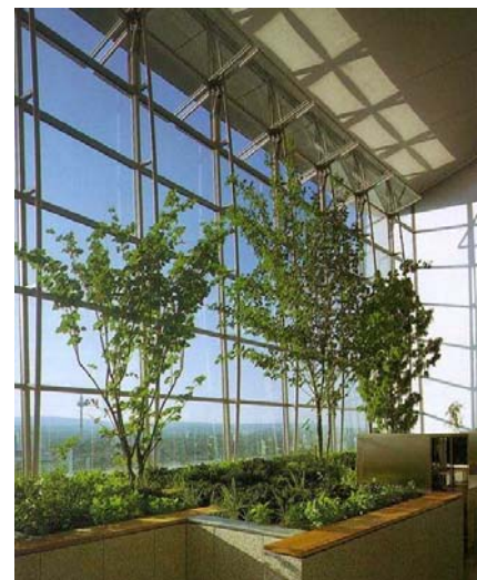
Fig. 40: Cavity with a width > 2000mm (atrium) Commerzbank (Frankfurt)
