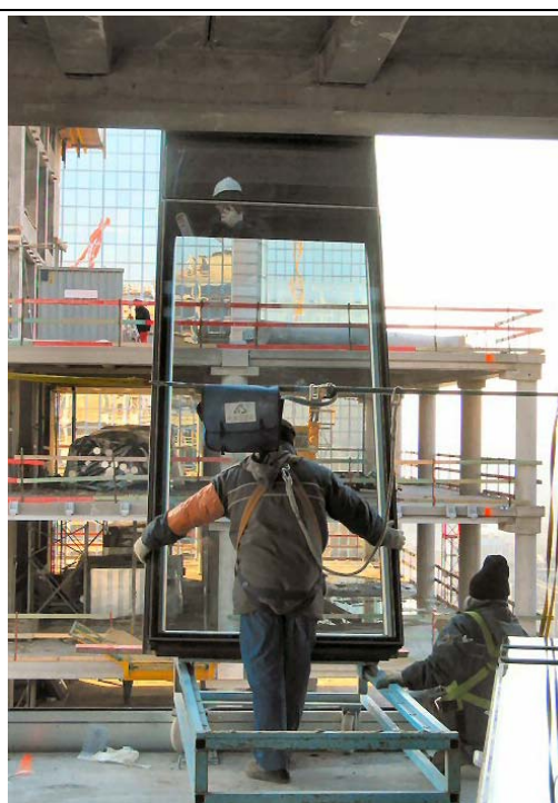
Fig. 4: Mounting of a mechanically ventilated double facade - curtain facade element - active facade partitioned by storey with juxtaposed modules
