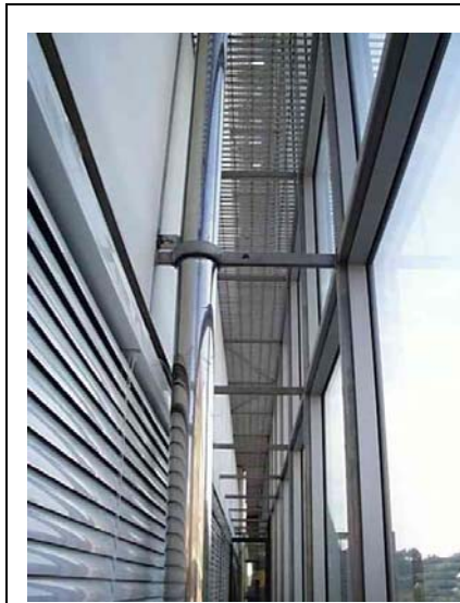
Fig. 7: Multi-storey ventilated double facade
