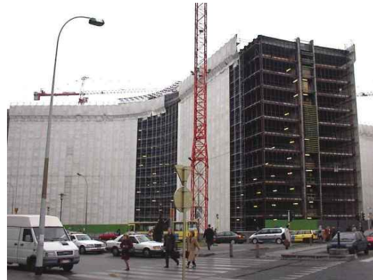
Fig. 27: Complete retrofitting of an existing building : Berlaymont (Brussels)
