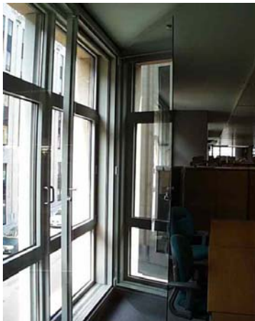
Fig. 32: Airtight indoor façade (can only be opened for maintenance reasons) DVV – Brussels
