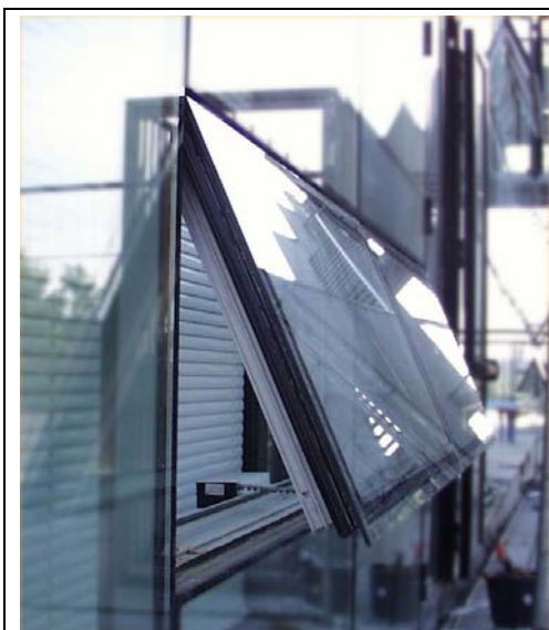
Fig. 12: example of motorised opening in a naturally ventilated double facade permitting the shift from one ventilation mode to another
