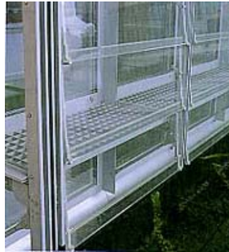
Fig. 37: Outdoor façade not airtight (cannot be tightened) Debis building (Berlin)
