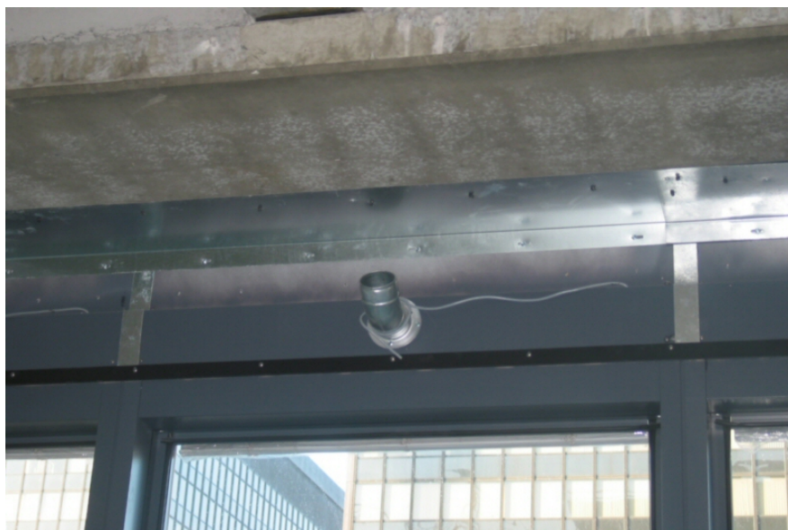
Fig. 15: View of the ventilation plenum linking a facade module to the building's ventilation system (to be connected)
