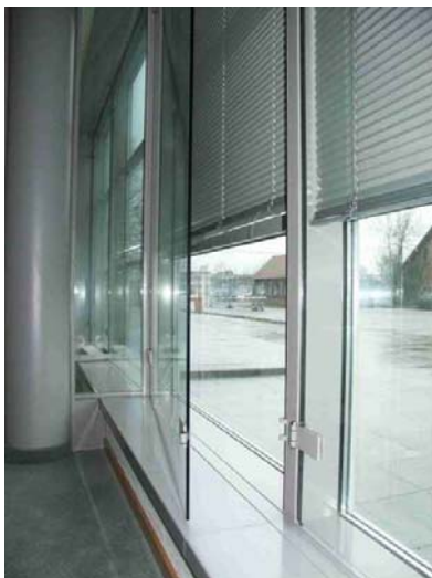
Fig. 38: Cavity width : 50...200mm (in this case Climate façade) UCB Building (Brussels)
