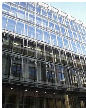
Fig. 35: Airtight outdoor façade (can partly be opened for maintenance reasons) Brussimo Building (Brussels)
