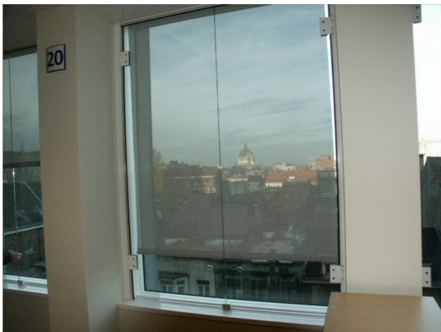
Fig. 17: Interior view of a mechanically ventilated double window – indoor air curtain ventilation mode
