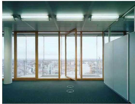
Fig. 31: Airtight indoor façade (can be opened by the user and for maintenance reasons) Düsseldorf city gate (Düsseldorf)
