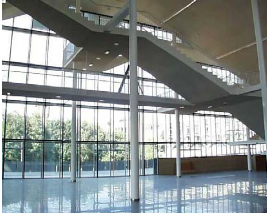
Fig. 30: Airtight indoor façade (cannot be opened even for maintenance reasons) Aula Magna (Louvain-la-neuve)
