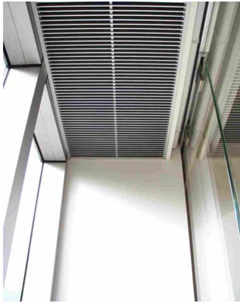
Fig. 19: View of a large cavity of a mechanically ventilated double facade partitioned by storey
