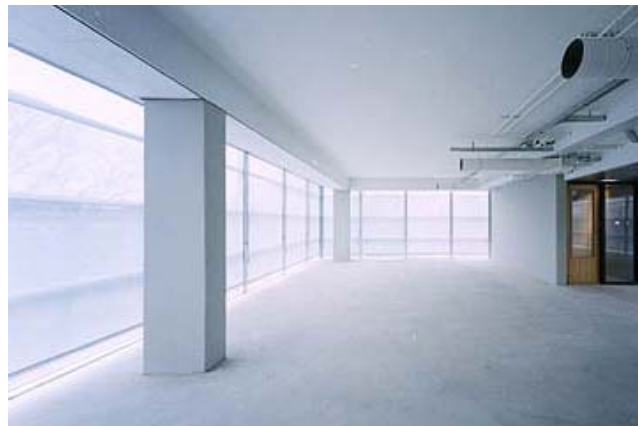
Fig. 33: Indoor façade not airtight (cannot be tightened) – in this case of a solar control serves as inner layer Mercator building - Nijmegen
