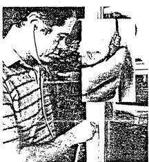
Checking for air leaks can be done with hollow-tube earphones (inset). When using simple tools like this, it's best to pick a day when it's quiet outside.
