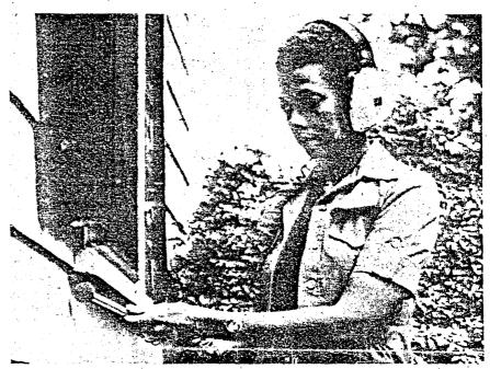
Detecting air leaks with a microphone and headset is done with a loud source of sound inside. Even small holes transmit about twice as much sound as the wall
