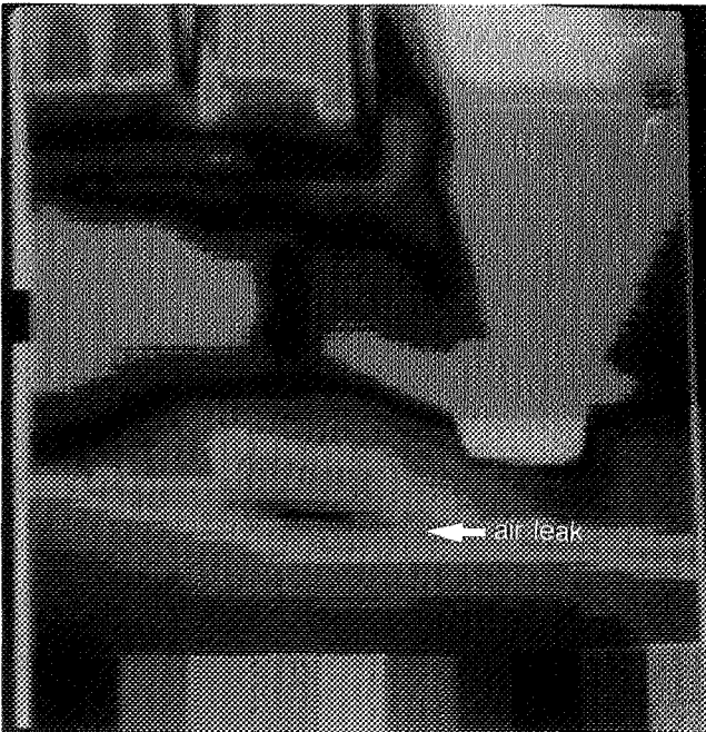
Figure 4b. Wall/floor interface while pressurized.
