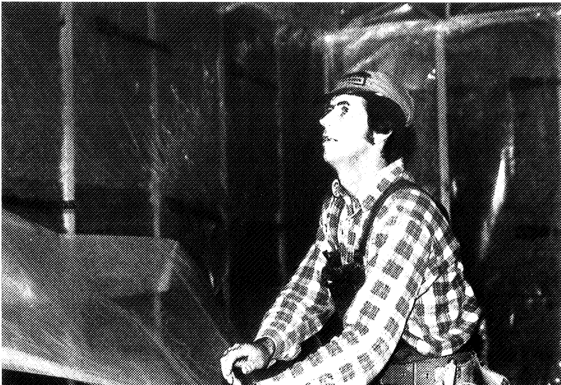
Figure 106. Large sheets of plastic foil are used so that the number of joints is kept to a minimum. The width of the foil is the same as the room height plus an extra amount for overlapping.
