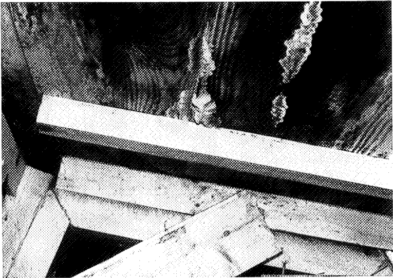
Figure 9. Blueing and initial rot damage on the roof panel. It can be seen that the main cause is the air leakage which can occur as shown in figure 8. Experience has shown that it is not possible to avoid damage by improving ventilation. Only by making joints airtight is it possible to eliminate moisture accumulation and the consequent risk of mould and rot damage.
