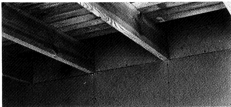
Figure 101. The plastic foil is clamped with the help of plasterboard sheets between the joists. To improve the airtightness further, sealing compound can be used adjacent to the joists.
