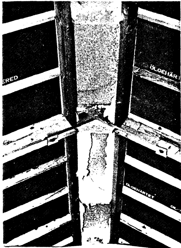
Fig 2 Capped ridge partially blocked by snow
