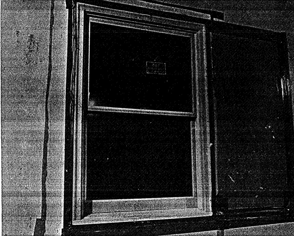
Figure 7. Wood double-hung window installed in filler wall.
